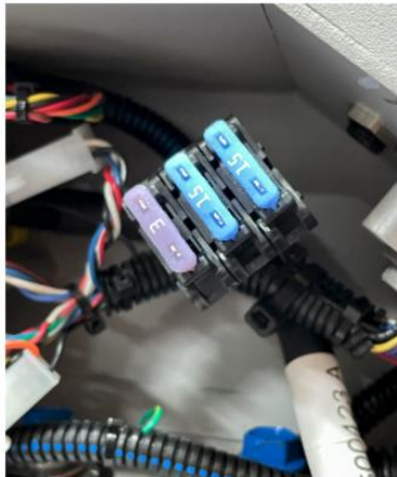
Figure 1: Fuse block with all 3 fuses in place
