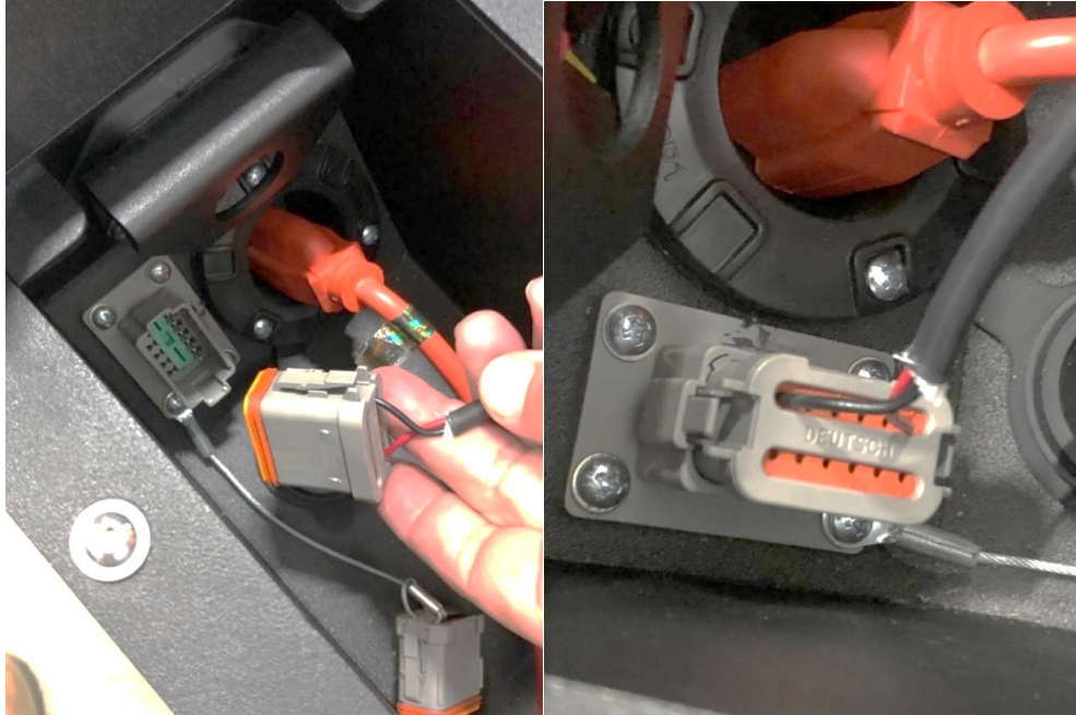
Figure 10: Connecting the jumper to the battery
