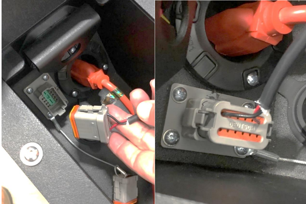
Figure 14: Connecting the jumper to the battery
